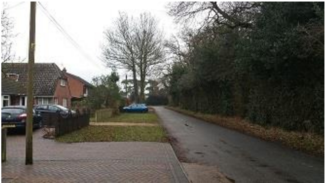
Figure 5: Overhead UKPN cable along road
