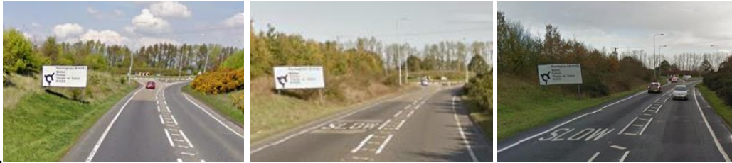
Images 2,3,4: View looking north at Colchester Road Roundabout 2009, 2012, 2015
