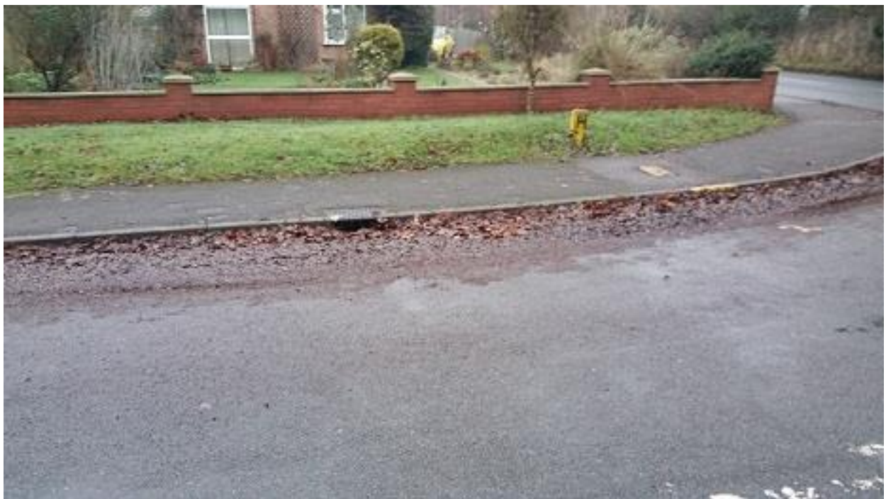
Figure 8: Existing kerb outlet on road
