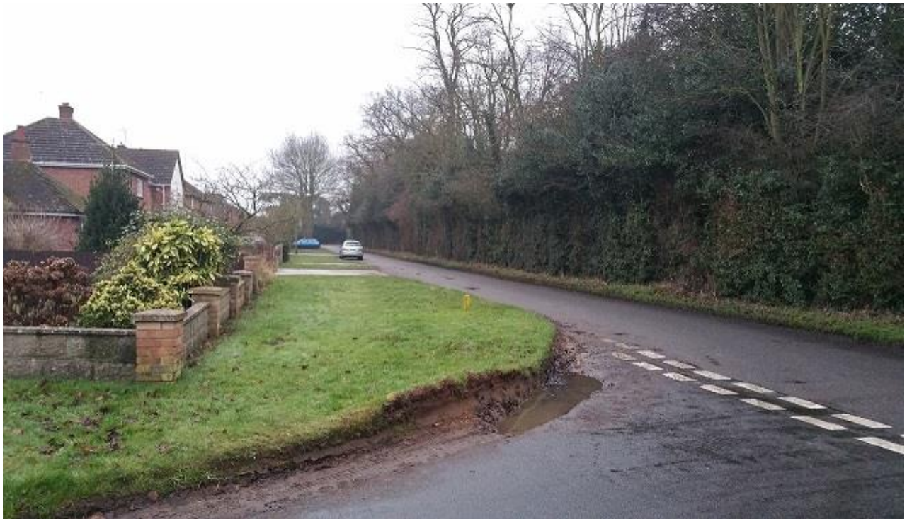
Figure 2: Verge damage due to vehicular over run and water pooling on road
