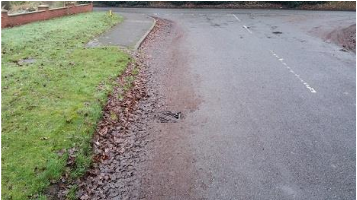
Figure 7: Existing gully on road
